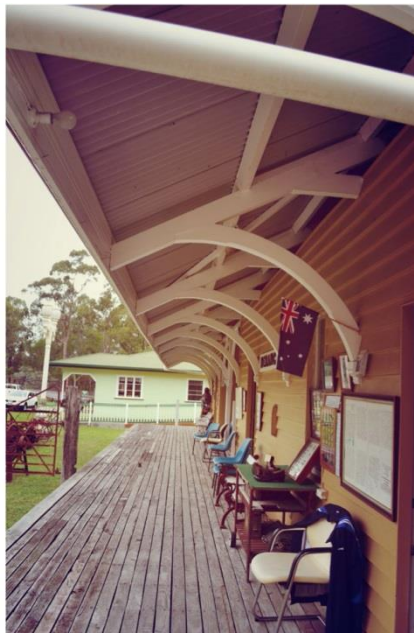
Fig. 10 (Right) Nerang Station waiting area, 2014
