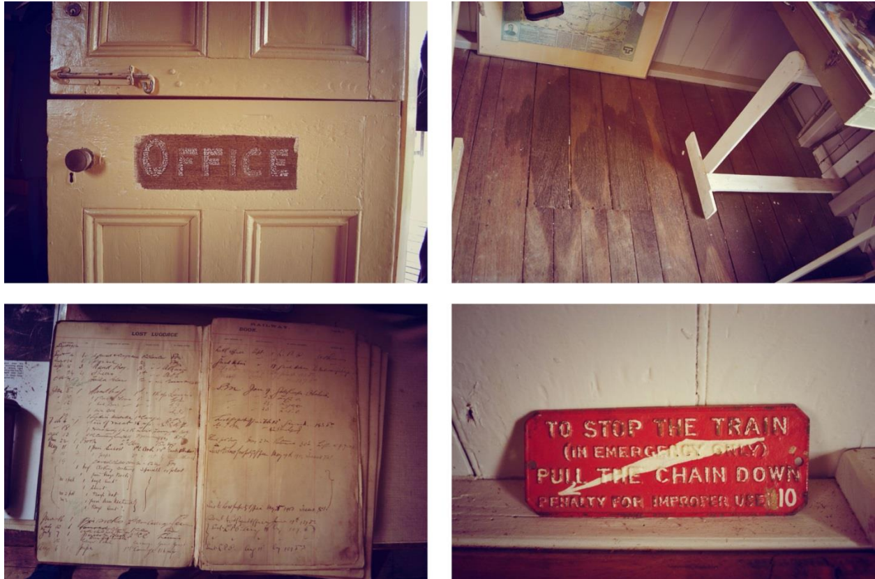
Fig. 12 – 15 (Top Right/Clockwise) Patched Lever Frame Hole, Emergency Stop Sign, Lost and Found Luggage Register, Station Master's Office, 2014
