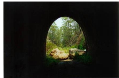
Fig. 33 Looking west out of Ernest Junction Tunnel
